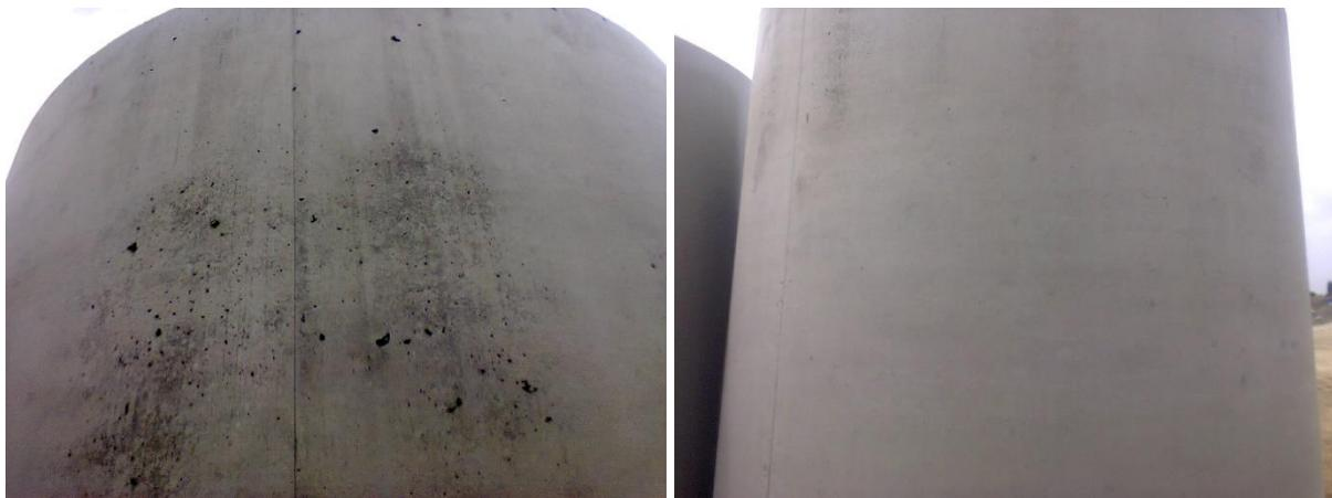
**Figure 1 Concrete segment surface finish with conventional concrete**
