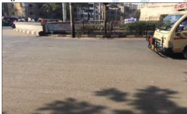
Figure 18 No zebra crossing at Model Town Intersection
